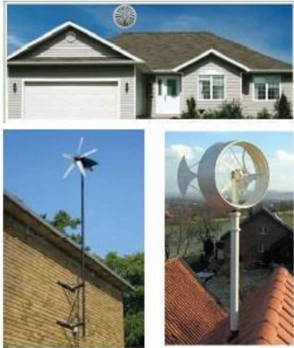
Figure 3: Examples of wall-mounted and roof-mounted Residential Scale Wind Energy Conversion Systems (RESWECS)
