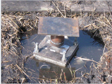
Installed Diamond Pier
