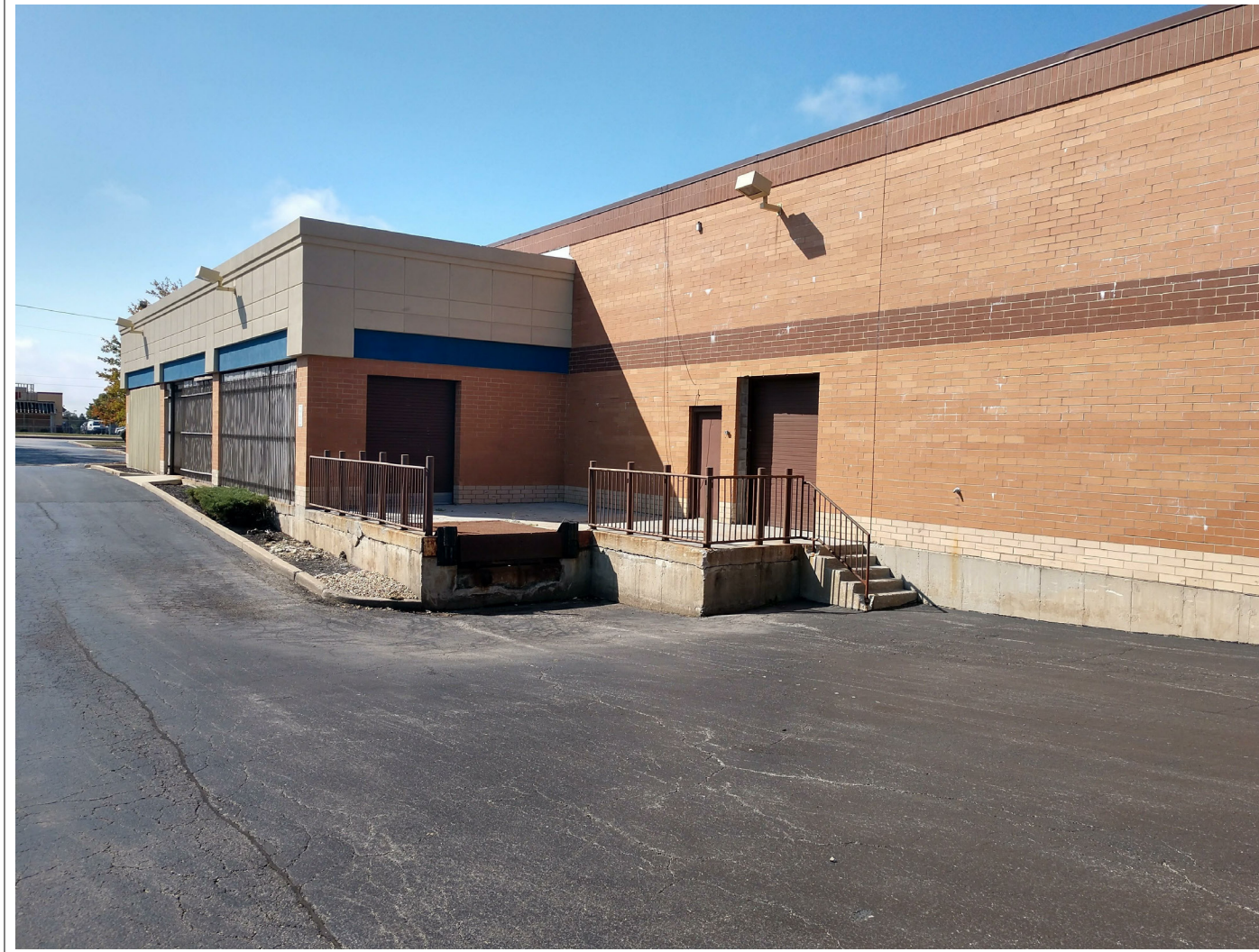
EXISTING CONDITIONS (DOCK AREA, LOOKING SOUTHWEST)
