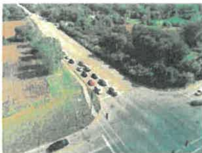
Looking West at the Dry Land Bridge
