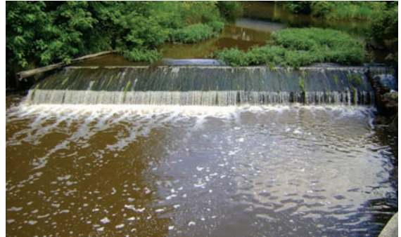
Spring Creek Dam at Draper Avenue, Joliet
