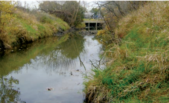
Straightened channel, Union Ditch at 191st Street, Tinley Park
