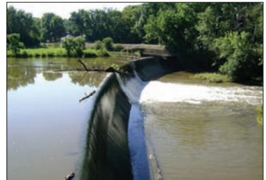
Dam on Hickory Creek at Pilcher Park
