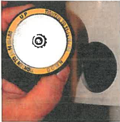
Figure 17 Placing rubber plug over access hole
