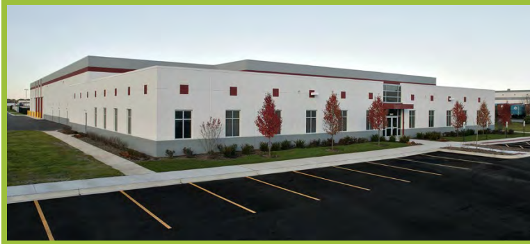
Village of New Lenox - Public Works Facility
