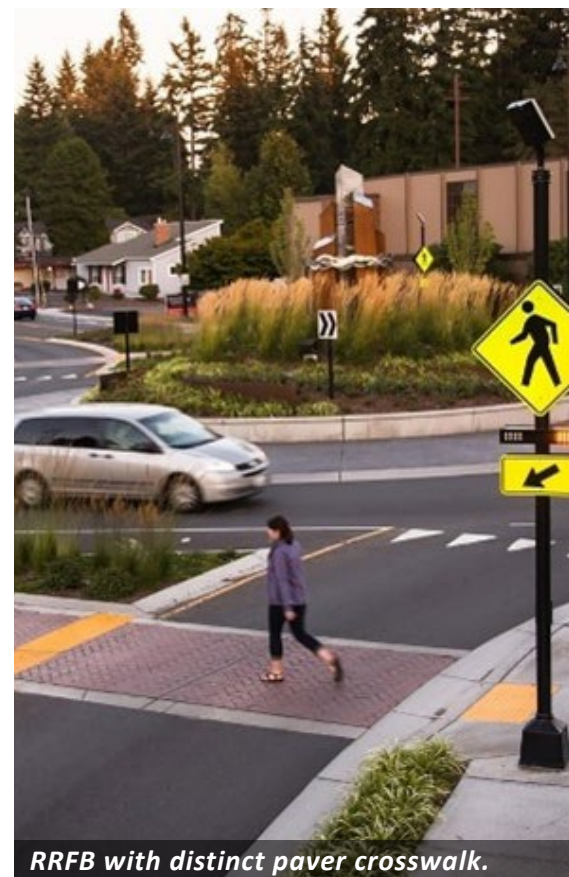
Pedestrian-Actuated Warning Beacon.
